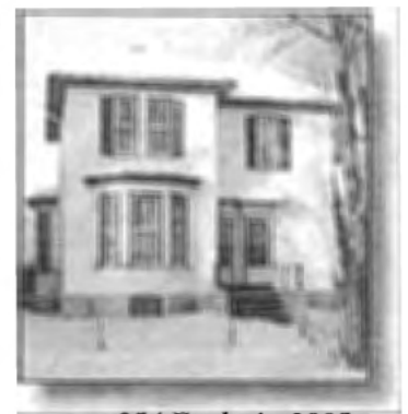
254 Furby in 2005: This is the oldest house still standing on the block.
