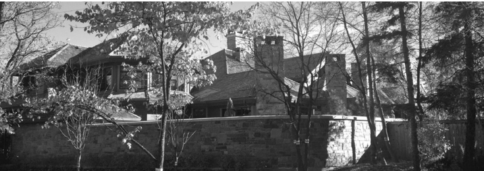
Fortress Winnipeg (2014): High walls surround this home in Old Tuxedo near Assiniboine Park.
